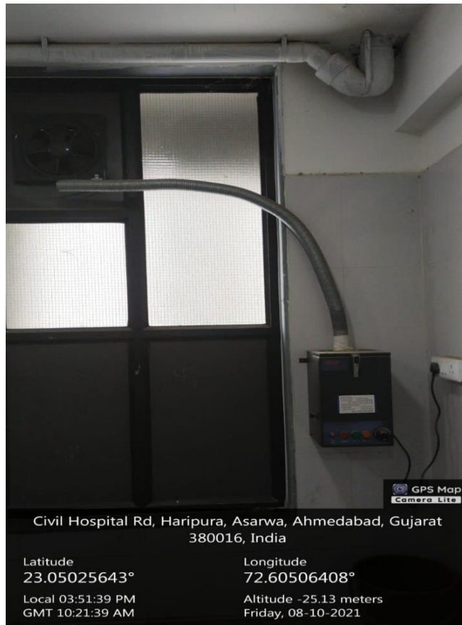
Electrical sanitary pad incinerator
